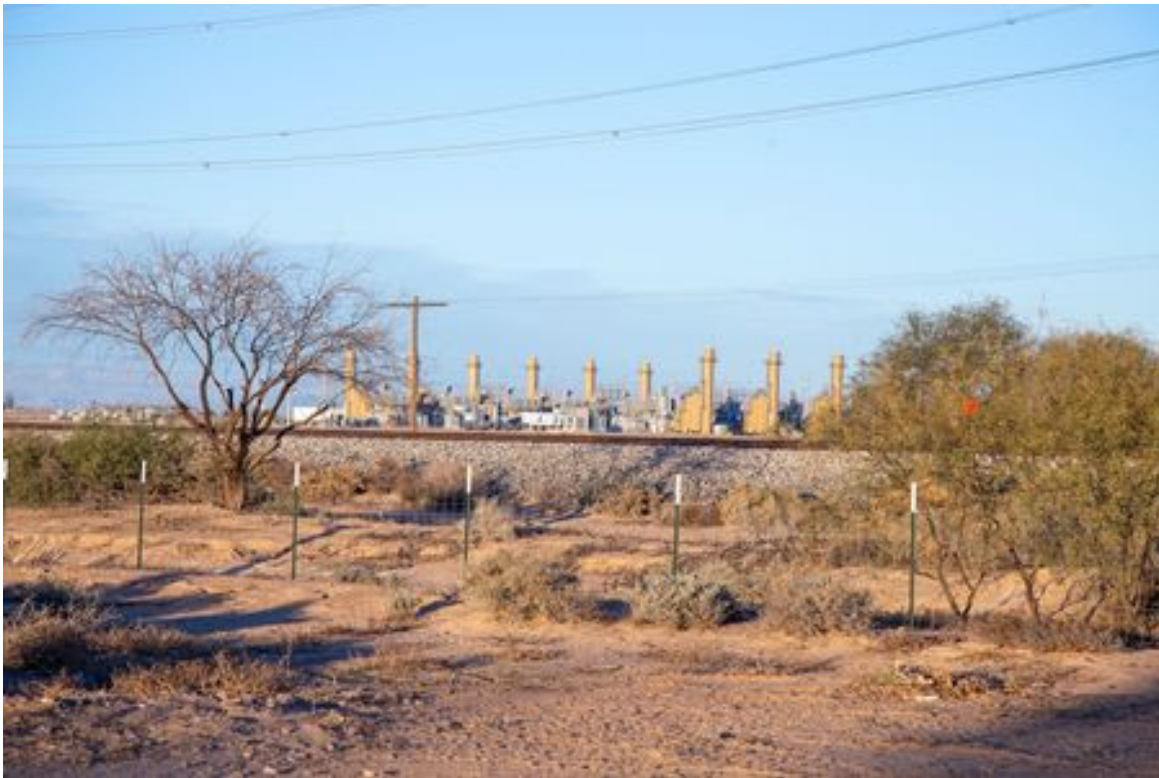
Coolidge Generating Station photo by Caryn Potter
