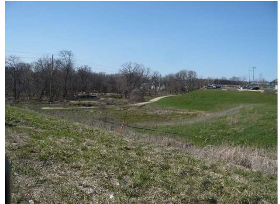
A parking lot and building built on a filled wetland next to Indian Creek in Marion, Iowa.
