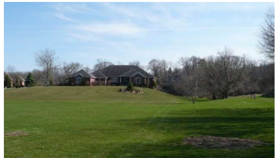
A house built on filled wetland next to Indian Creek in Cedar Rapids, Iowa.
