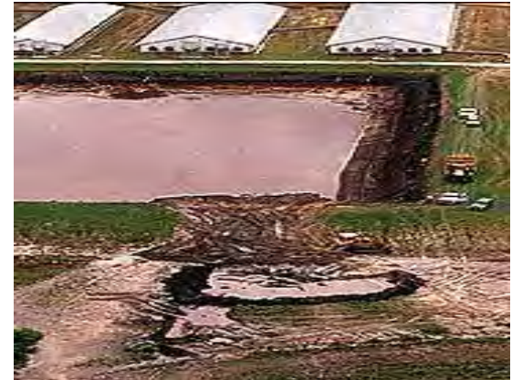
Lack of proper operation and maintenance results in a failed berm.
