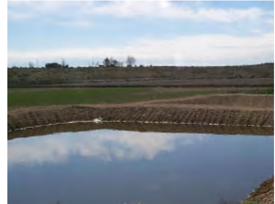
Well maintained earthen lagoon facilitates proper operation and maintenance.
