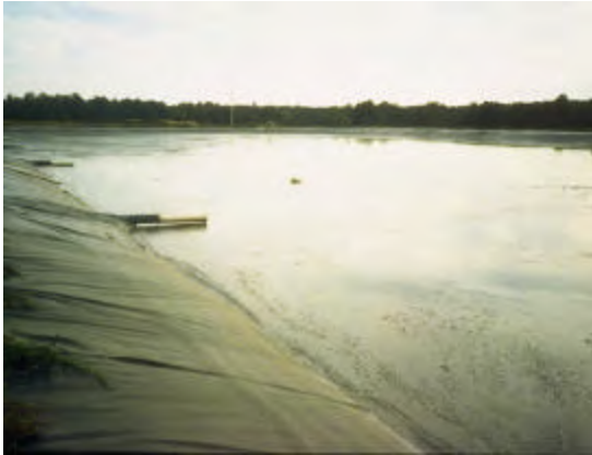
A lined lagoon with adequate storage capacity protects ground and surface water.
