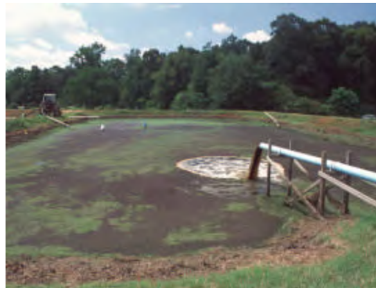
Undersized and poorly managed lagoon.
