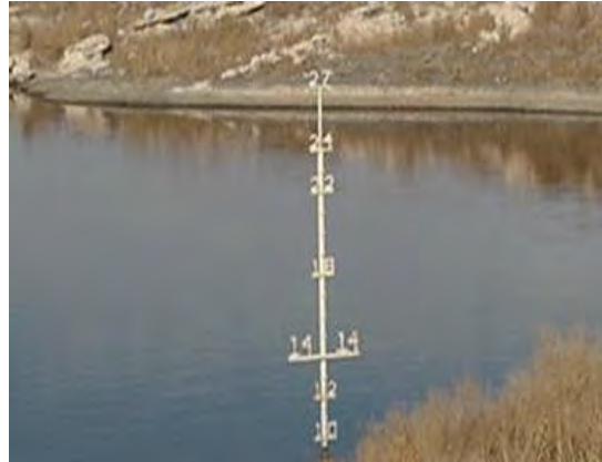
Depth markers gauge wastewater levels and help avoid capacity issues.
