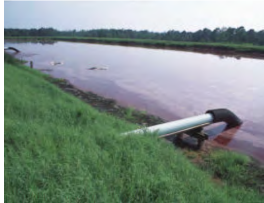
Waste deposited under the surface of a lagoon could help reduce offensive odor.
