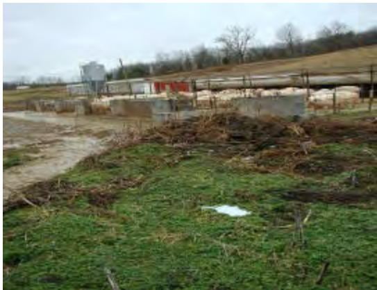
Poorly designed and maintained facility.
