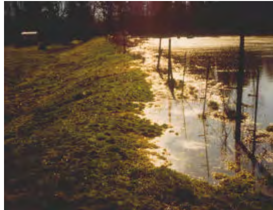
Overflowing lagoon has exceeded its capacity.
