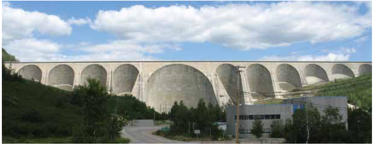
Hydro-Quebec's Barrage Daniel-Johnson Dam on the Manicouragan River in Quebec Province.
