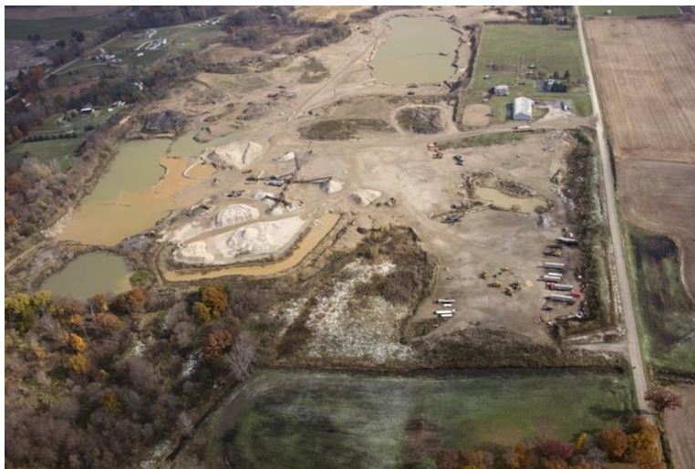
Sand and gravel mine in Grass Lake Twp showing lake created in violation of state environmental law (top of photo)
