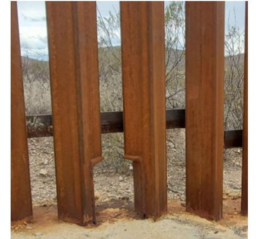
Example of a small wildlife passage at the wall. Photo by Erick Meza
