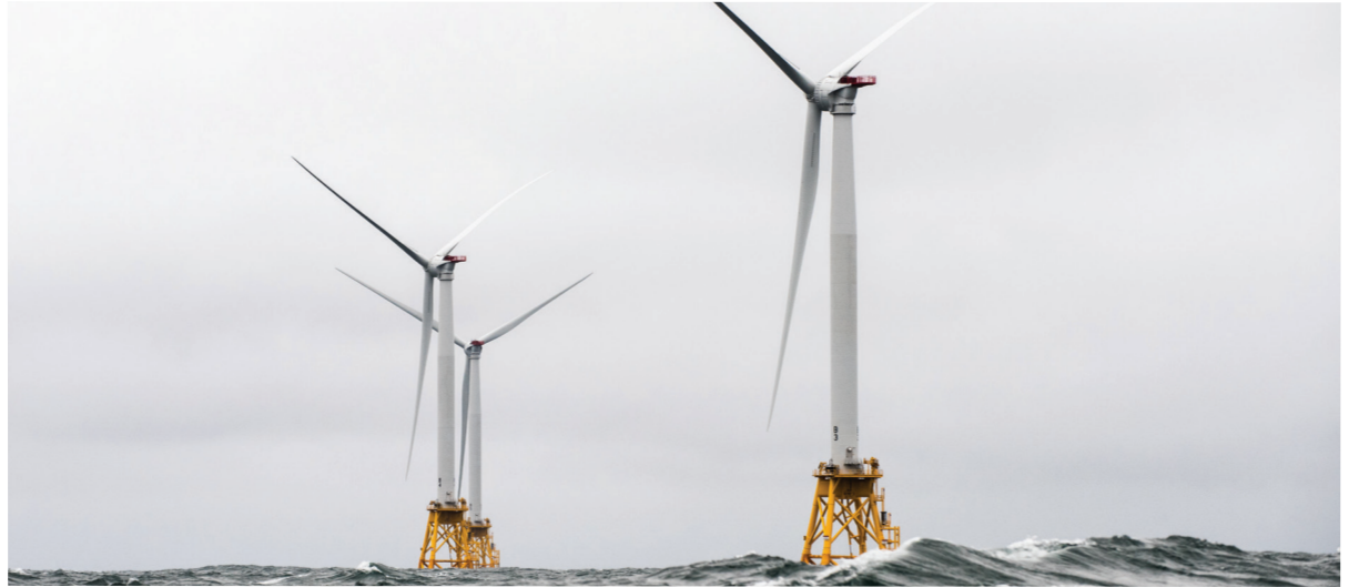
Photo by Dennis Schroeder, National Renewable Energy Laboratory 40389
