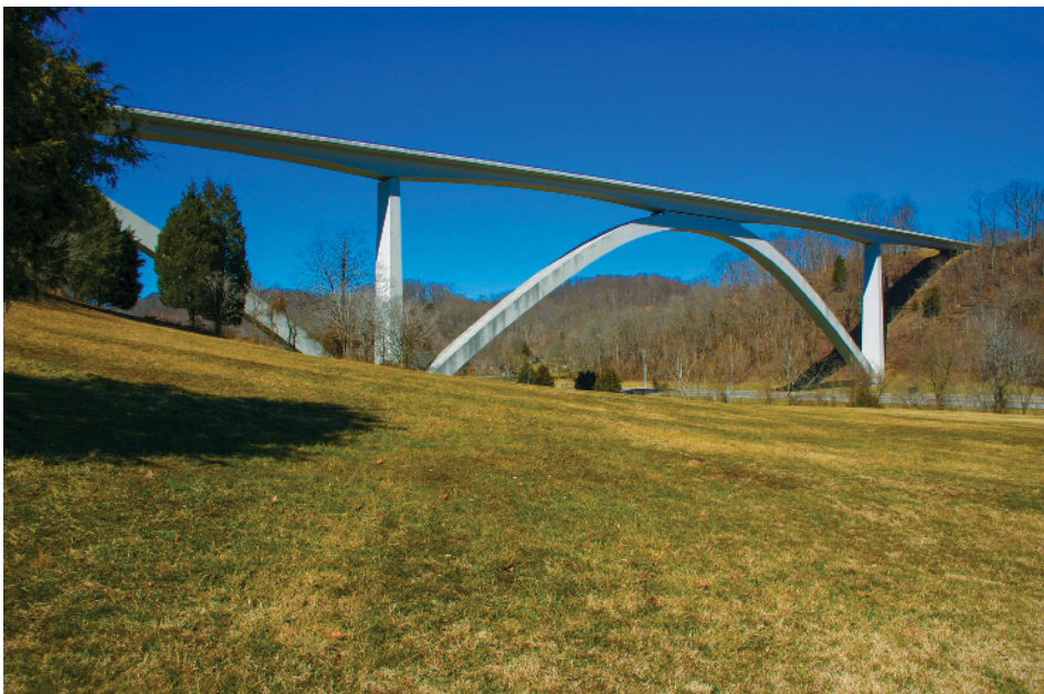
The Natchez Trace Parkway Bridge is a concrete, double-arch bridge located in Williamson County, Tennessee, 8.7 miles from the northern terminus of the Natchez Trace Parkway. It is 1,572 feet long and carries the two-lane Natchez Trace Parkway over State Route 96 and a heavily wooded valley. Photo by Alan Sparkman.
