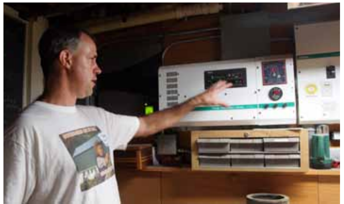
Solar Power Specialist and Master Electrician, Andrew Bangert explains the inner-workings of his home's solar system at an open house in August.
