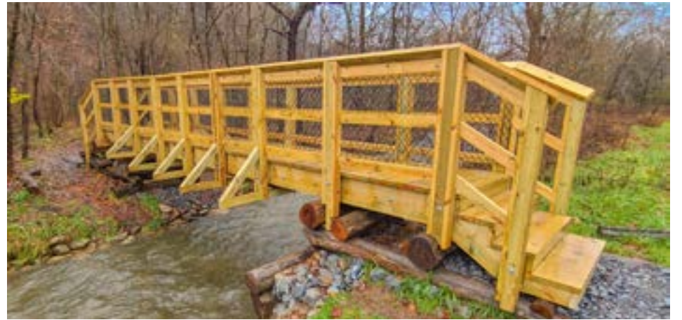
Jacob's bridge built by volunteers over Sinking Creek in Jacob's Nature Park, Johnson City, Tennessee.
