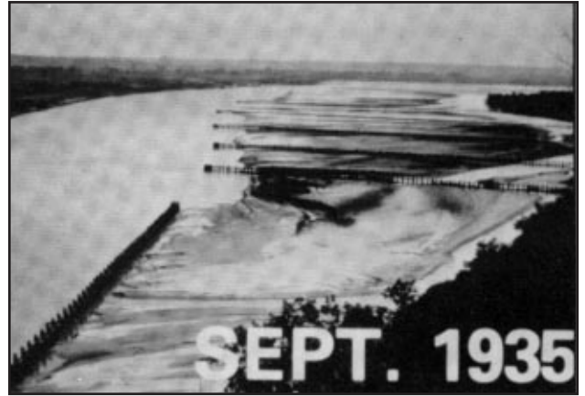
Figure 2.7 Changes in Channel Morphology Following the Addition of Navigation Dikes, Indian Cave Bend, Missouri River, North of Rulo, Nebraska.
