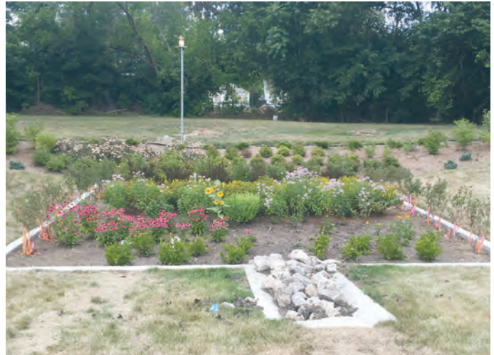
Bioswale promotes drainage.
