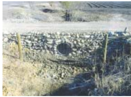
Much better The removal of a too-small culvert (above) freed the creek (below).
