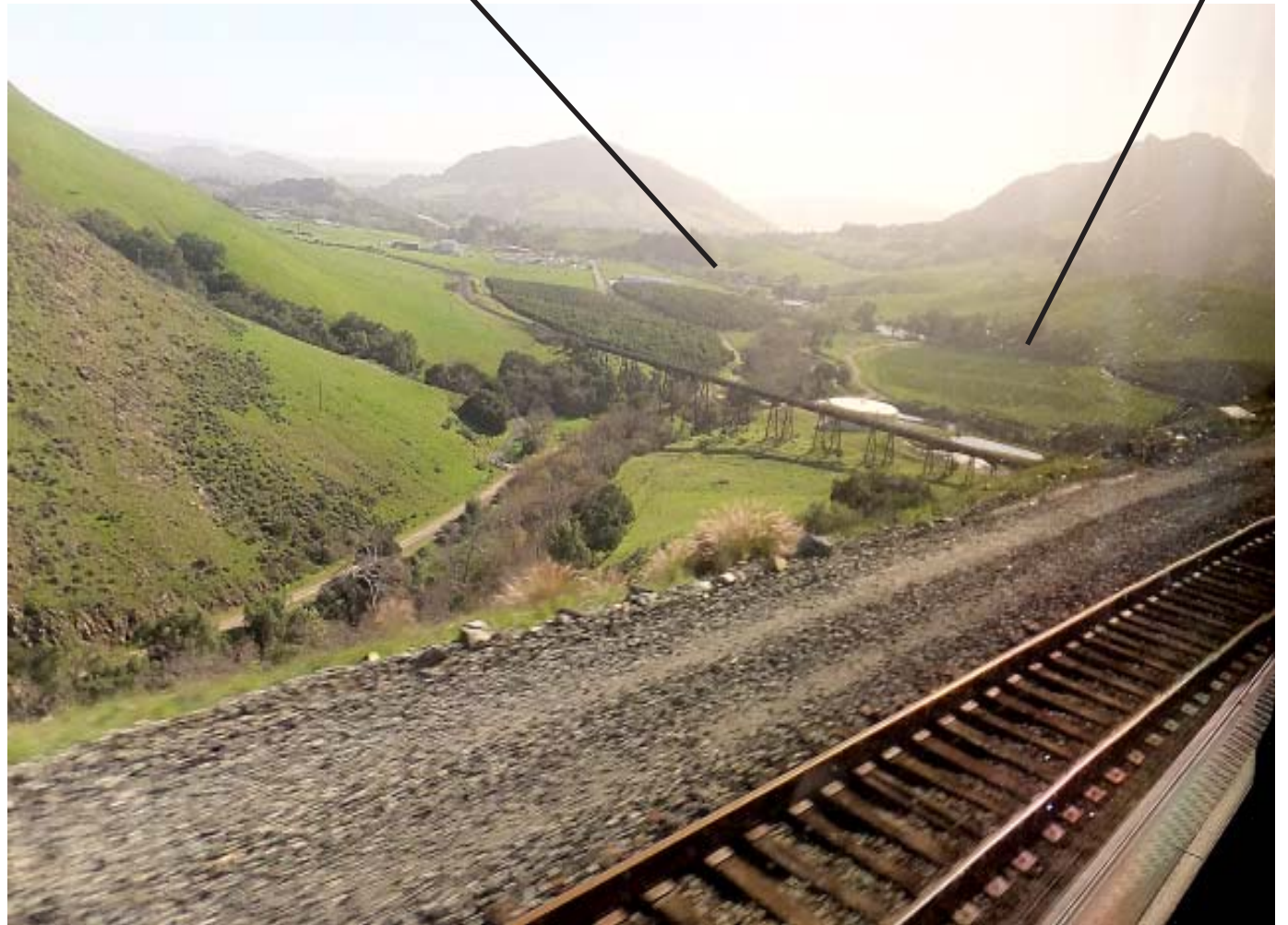
Fat target Every drop of the City of SLO’s main water supply -- from Santa Margarita Lake, Whale Rock Reservoir and Nacimiento Lake -- flows through the Stenner Creek Water Treatment Plant, located at the bottom of one of the most hazardous railroad grades in the state.
