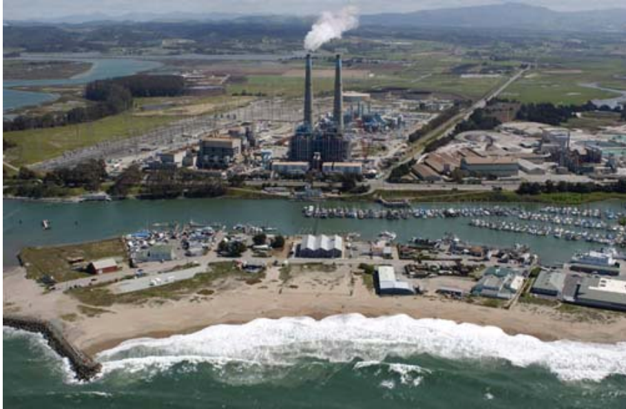
Moss Landing Power Plant/Cal-Am "test" Desalination Facility (December 2006)
