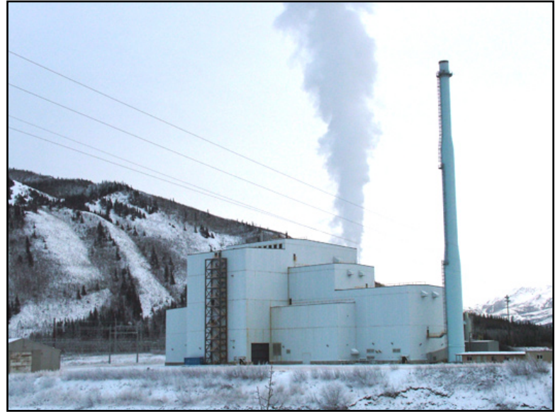
Healy Coal Plant #2 located in Healy, Alaska
