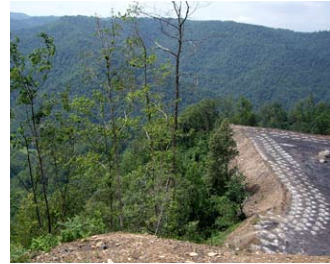
A series of "blast holes" where ammonium nitrate and diesel fuel is placed and ignited, sending rock and debris flying. People living as far as 12 miles from mining sites have reported hearing the blasts.
