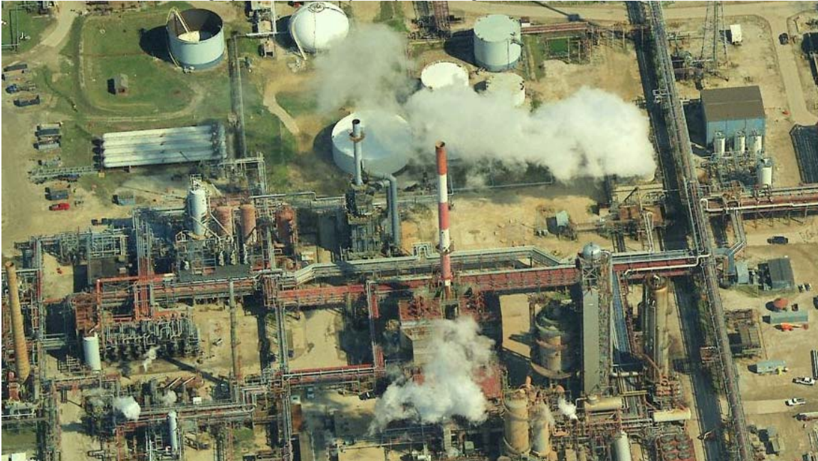
Below is an aerial image from BP's refinery in Oregon, OH.
