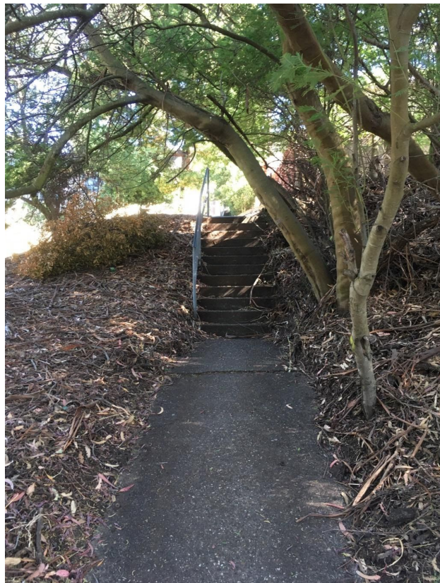
Second set of stairs from Drake to Park Circle
