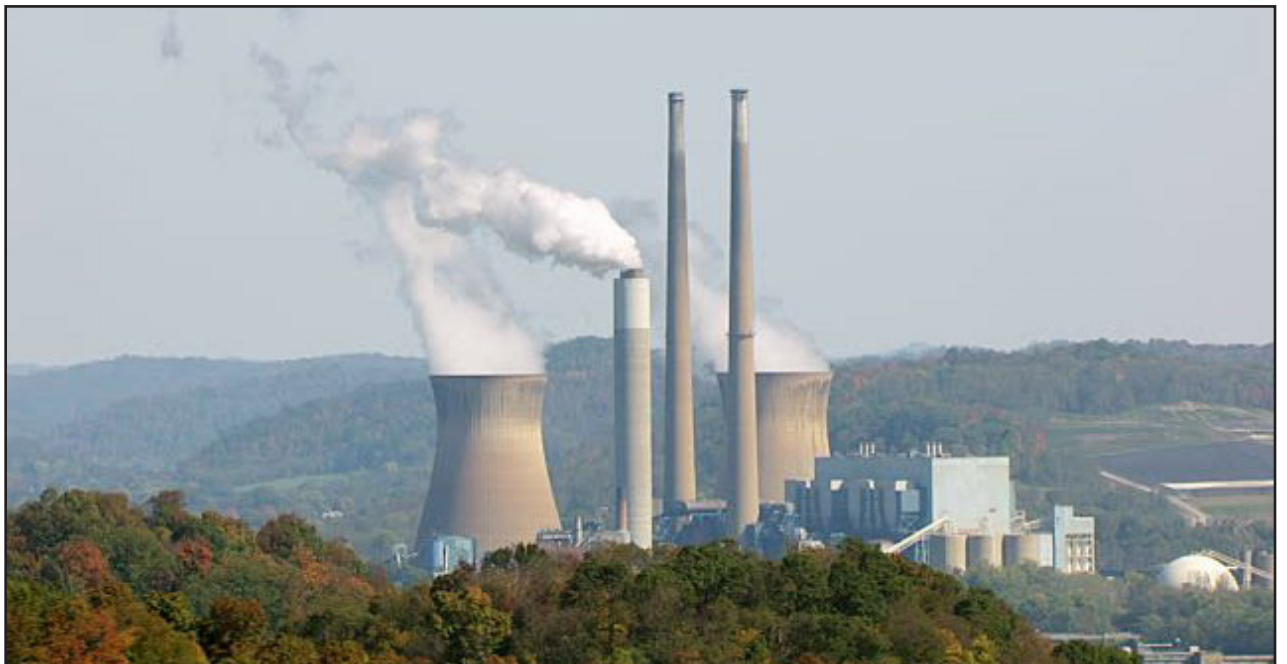
Pleasants Power Plant, Belmont WV
