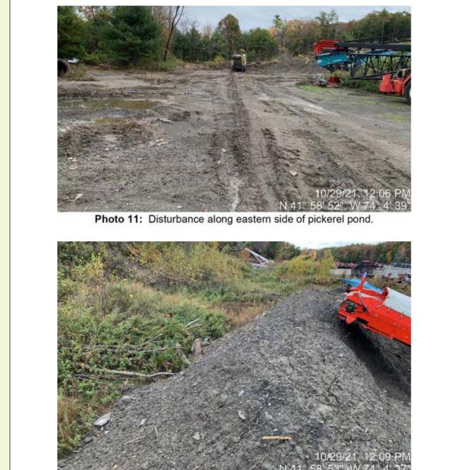
Photo 12: Material Stockpiles with no erosion controls.
