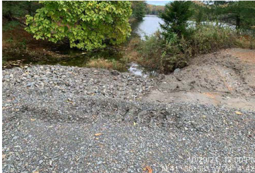
Photo 16: Fill Placed on bank of Pickerel Pond.
