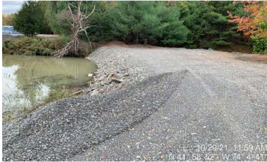
Photo 9: Fill Placed in Pond B and on bank of Pickerel Pond.
