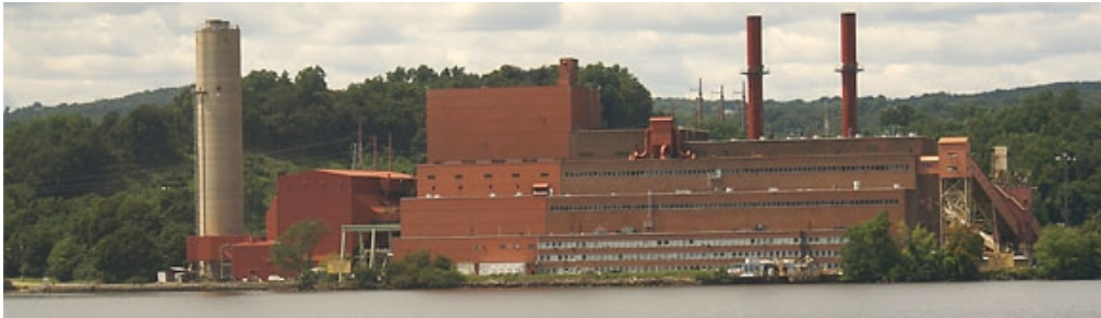
Danskammer Energy River Road facility
