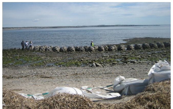
Reef balls, made of cement, at Stratford Point in Stratford, Connecticut, currently attempting to protect 750 feet of shore, by mimicking a natural oyster reef.
