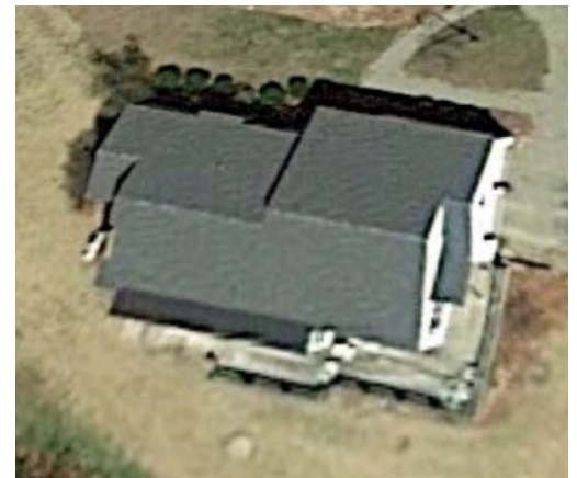
Long south sided roof, perfect for solar panels
