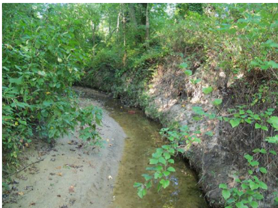
Eroded Stream Bed
