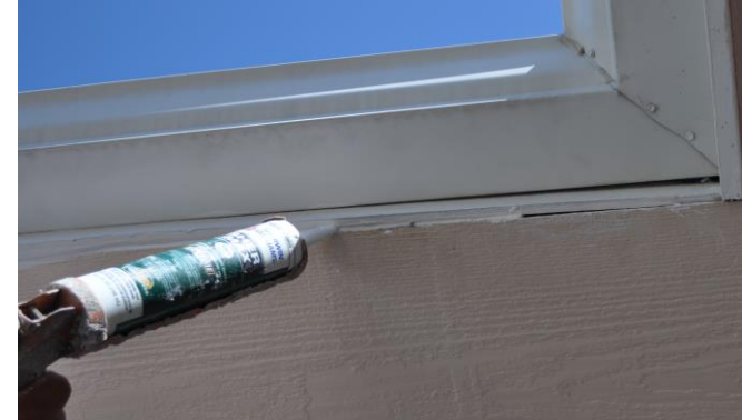
Caulk the interior trim
