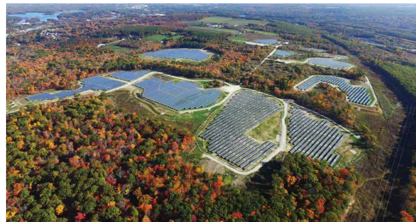
16.5 MW DC solar farm built in Oxford, MA. This 130-acre property was previously known as the largest pig farm in Massachusetts. Photo by Lucas Faria.
