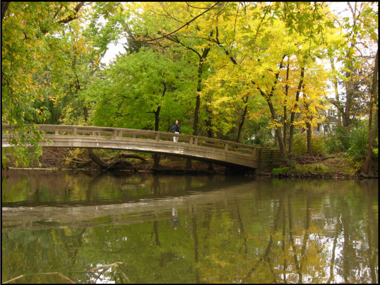
Figure 2. Reach 8 of ILD980823991, showing pedestrian bridge.
