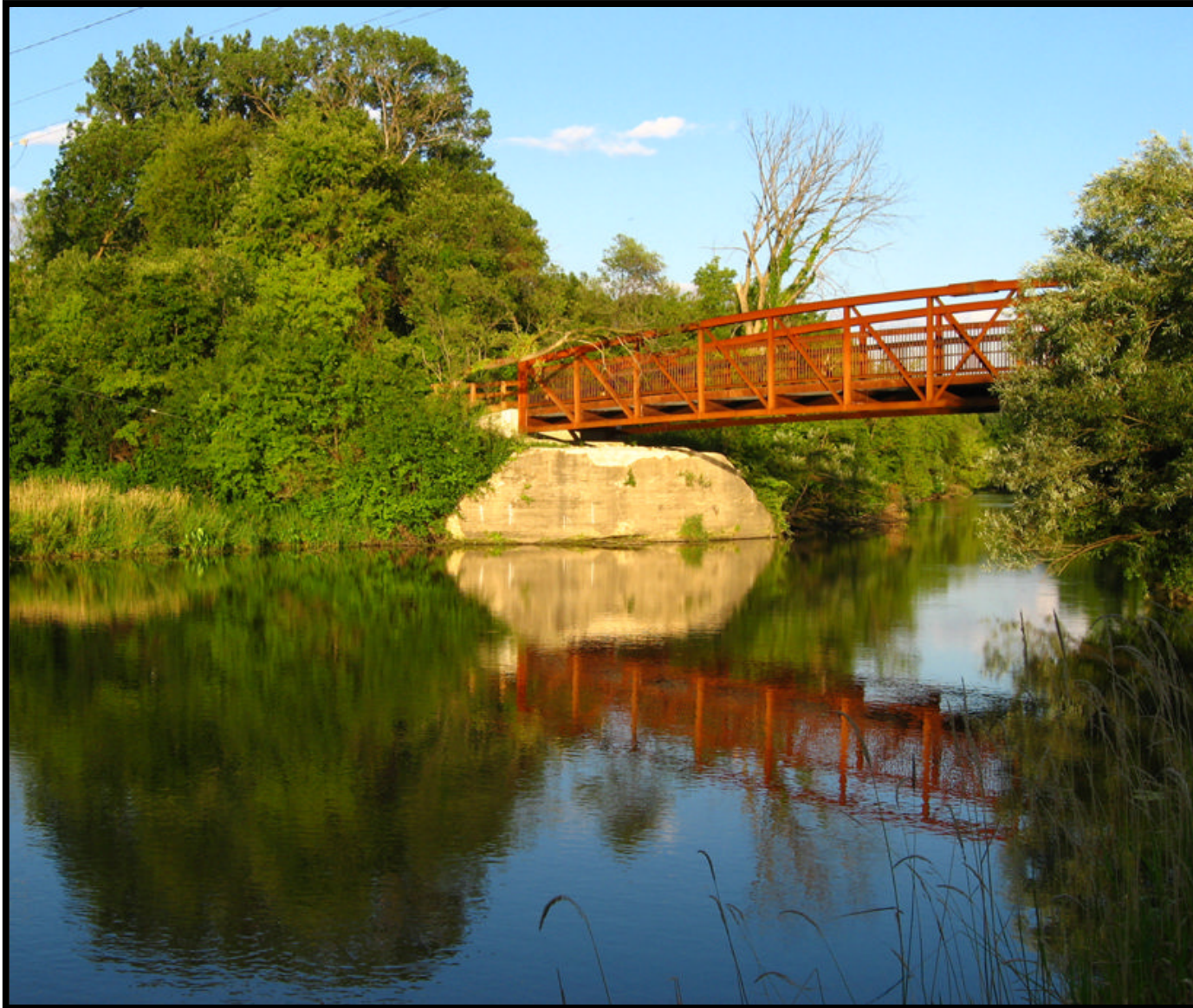
Figure 1. Reach 7 of ILD980823991, showing pedestrian bridge.
