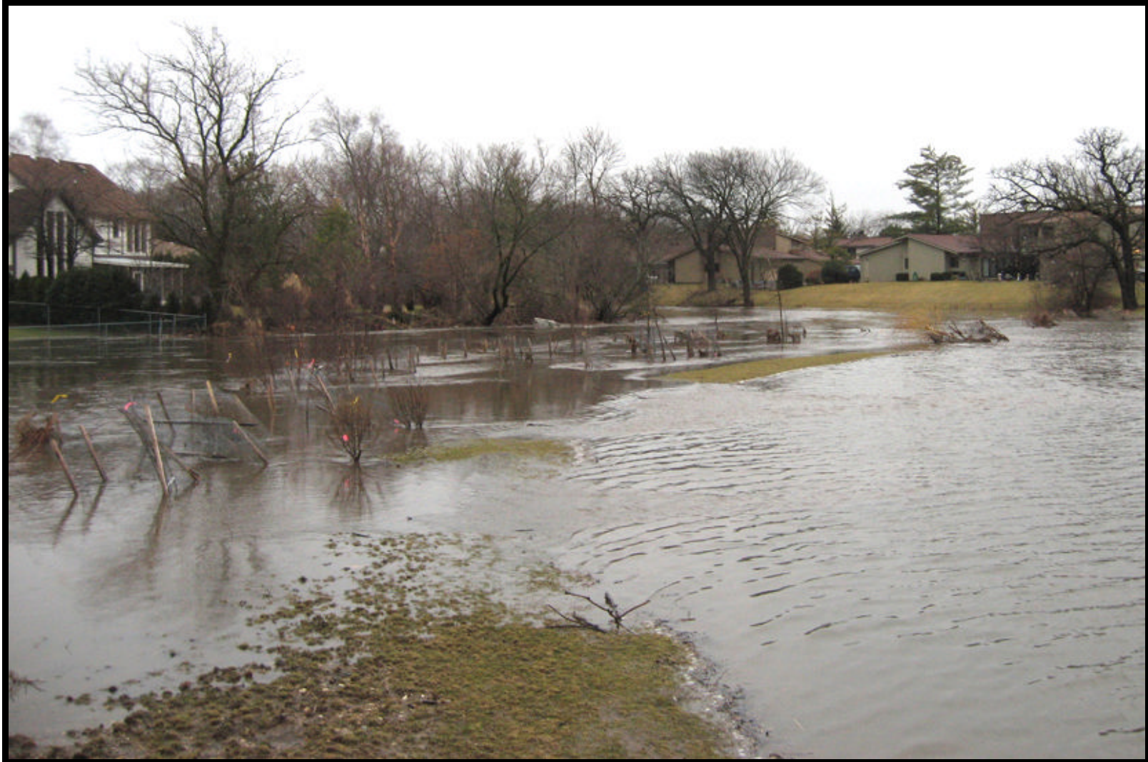
Figure 3. Reach 5E of ILD980823991 at floodstage. Note eroded, breached bank in foreground and destroyed restoration plantings along its entirety. Excavation completed 12/07, photo taken on 3/9/09.
