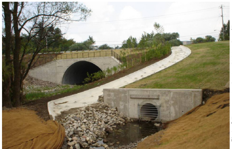
The Finch Avenue washout after an extreme precipitation event in Toronto 2005.
