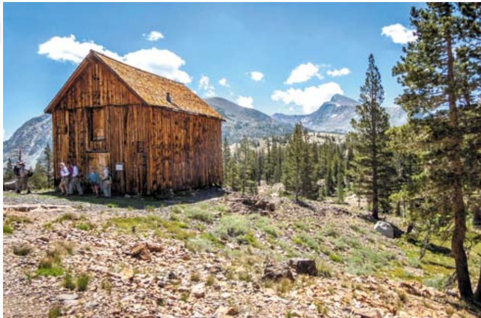
Bennettville: July 5, 2015. Tioga Pass Road was created to give access to the mine at Bennettville. On this overcast morning, Range of Light hikers went first to the old mine and then wound their way down to the remains of the town of Bennettville, which has only two buildings standing. Photo: Joanne Hihn.
