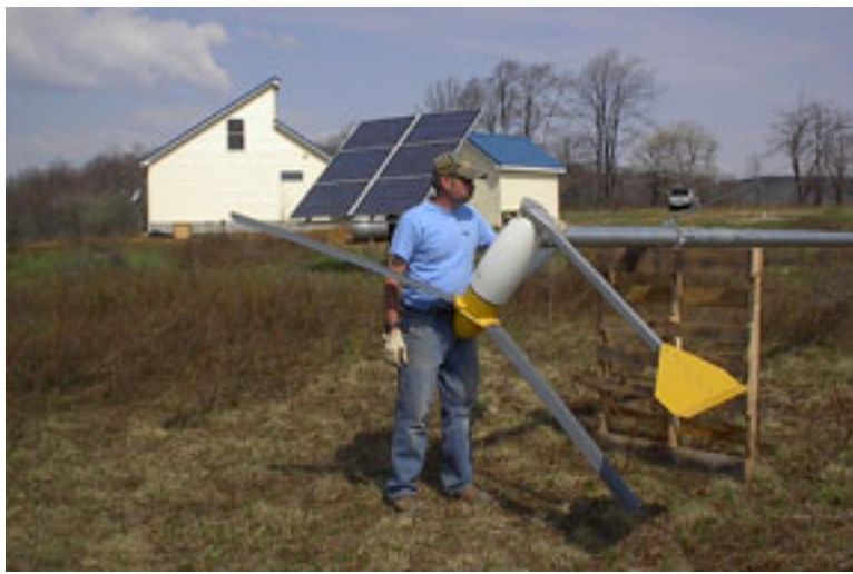
The windmill can be lowered for easy maintenance. Solar array and house are in background.
