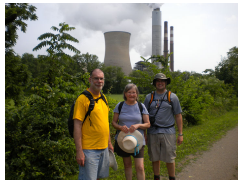
Hikers learn about Fort Martin Power Plant's new scrubbers on June outing along Morgantown Rail Trail.
