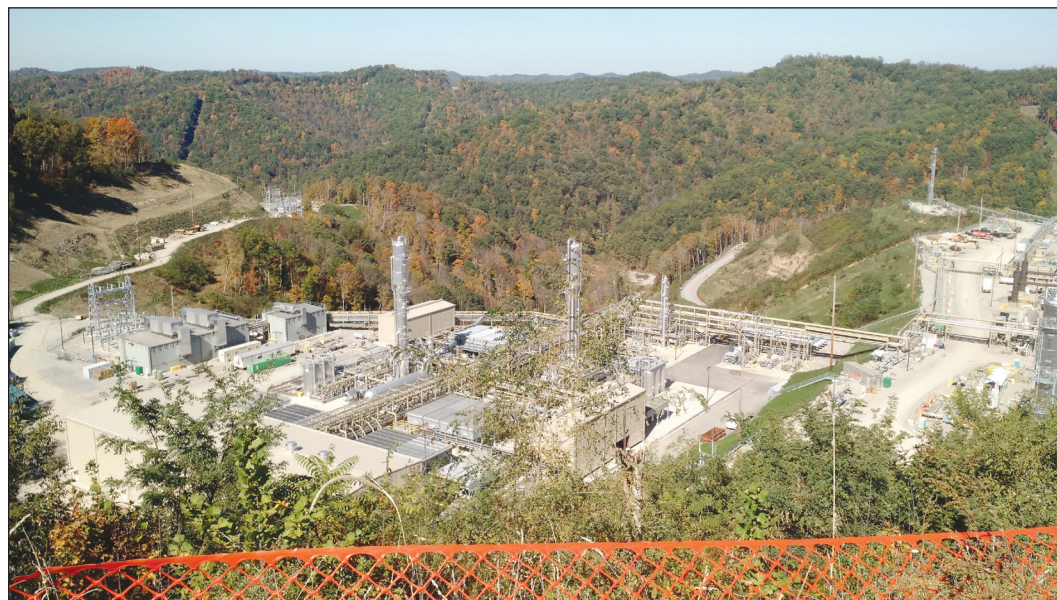
A stunning view of the huge MarkWest plant in Mobley.
