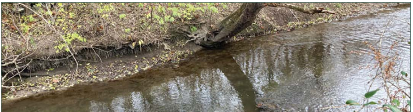
Evitts Run carries water between Charles Town Utility Board's sewage plant through Willingham Knolls Park (shown here) to the Shenandoah River. PHOTO BY LYNN DELLES.
