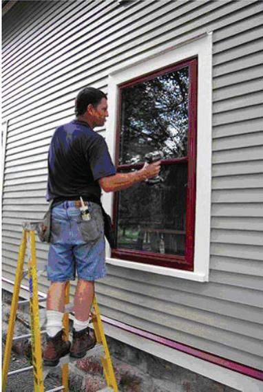
Storm windows with Low-E glass installed over original restored windows, creating a well-sealed secondary glazing
