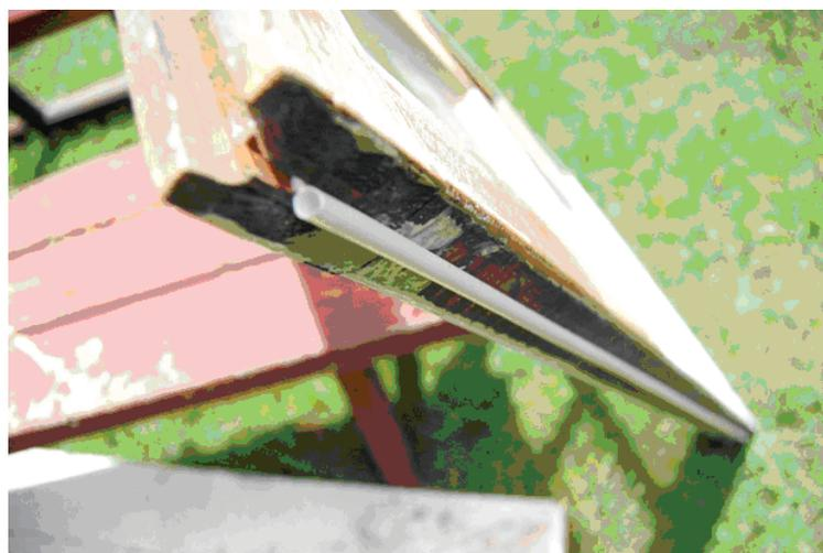
IMAGE 2: Silicone tube seals in kerf in the head of the upper sash, at the meeting rail of the lower sash, and at the sill of the lower sash.
