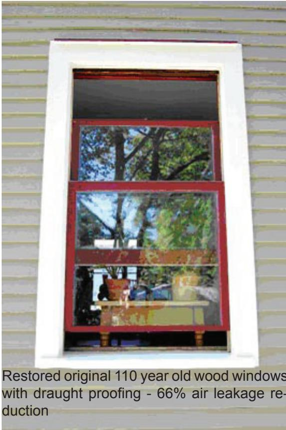
Restored original 110 year old wood windows with draught proofing - 66% air leakage reduction
