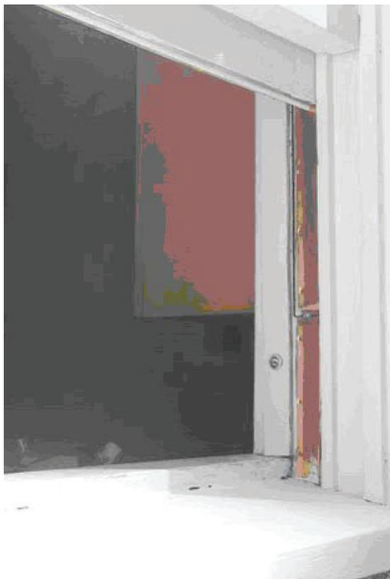
IMAGE 1: Bronze spring weatherstripping installed in both jambs.
