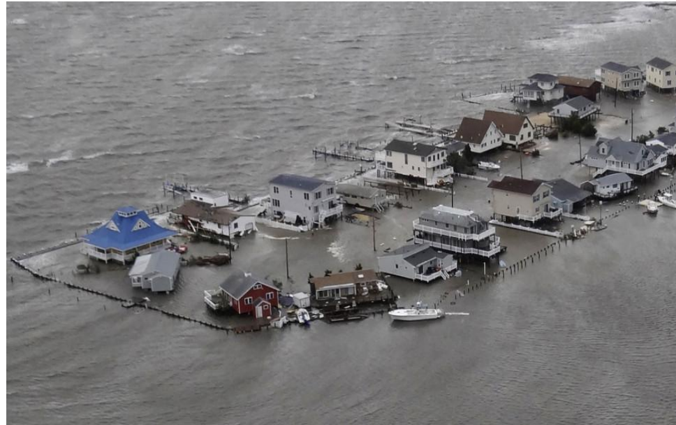
Flooding in Tuckerton during Hurricane Sandy, Photo by: CNN News
