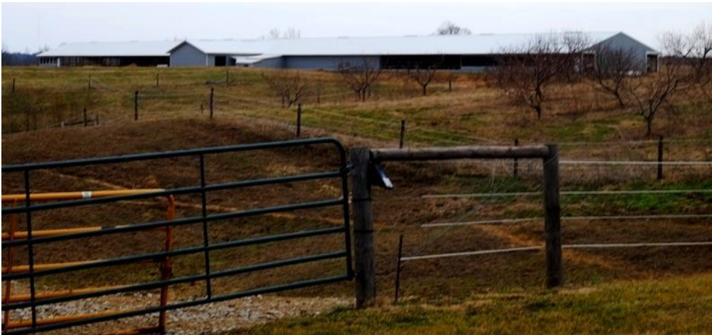
New chicken farm building uphill of northwest edge of Cedar Lake. Sabrina Hardenbergh, 2016
