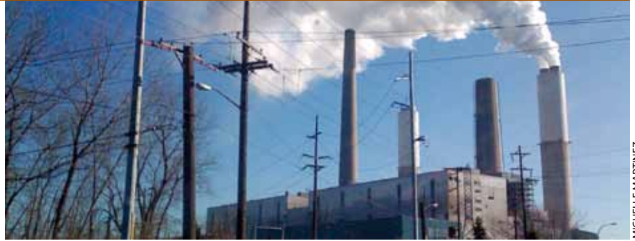
DTE Monroe Power Plant
