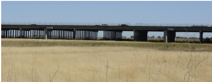
Box Girder Causeway
