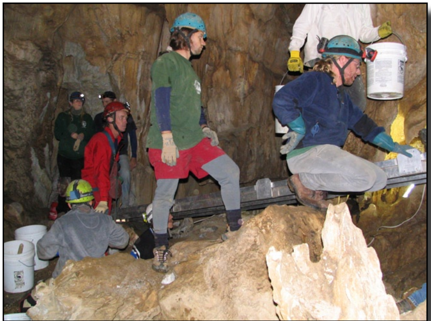
Installation of a bridge protects fragile formations in Crystal Cave.
