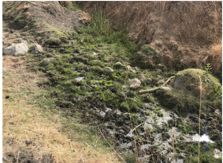
Figure 2: Waterways and wetland degradation, Coyote Lake County Park, Fall 2018
