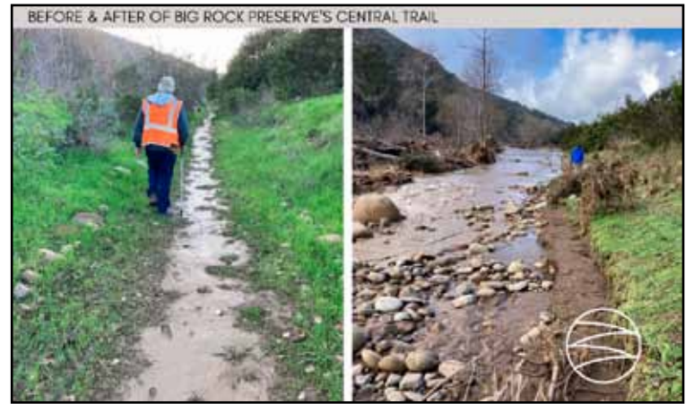
Before and after photos of Big Rock next to the Ventura River. All trails and recent plantings were washed away, so Ventura Land Trust has it closed for now, but if you'd like to volunteer bringing it back, go to:
