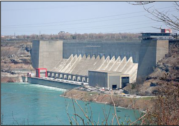
Robert Moses Niagara Hydroelectric Power Station photo: Creative Commons
