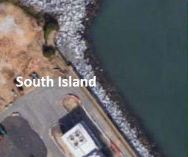
Rock revetment connecting both islands
