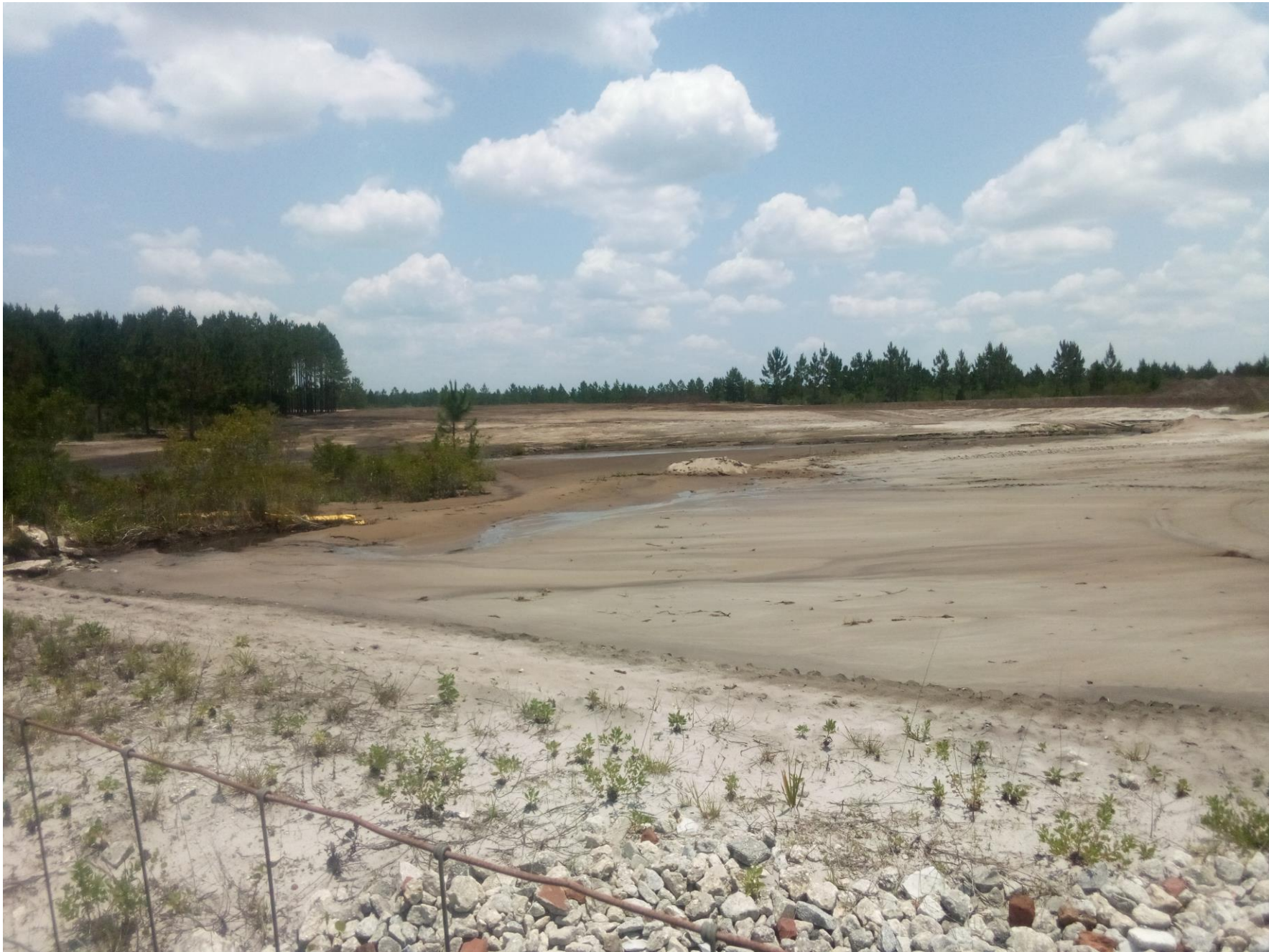
Reclamation underway June 2023
