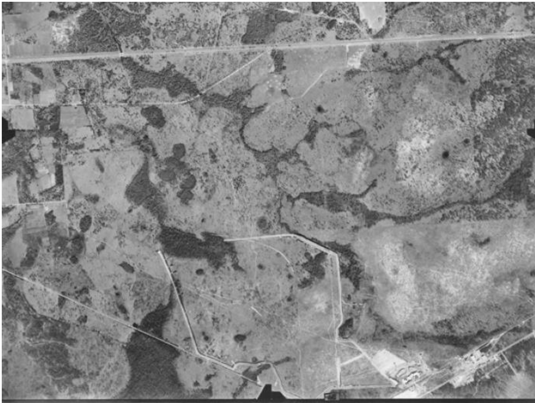
Pre mining in 1949 with the DuPont plant being constructed
