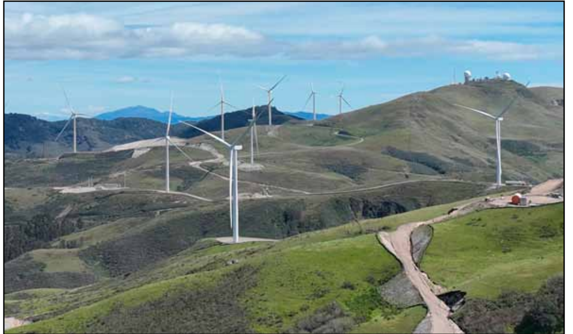
Thar she blows! Or will soon as the last of 27 wind turbines are about to be switched on in the hills south of Lompoc. This is a major stride in SB County's push for renewable energy and well-paid green jobs. Follow its status here: www.twitter.com/StraussWind (© Photo Gwendolyn Garcia courtesy of BayWa r.e.)
