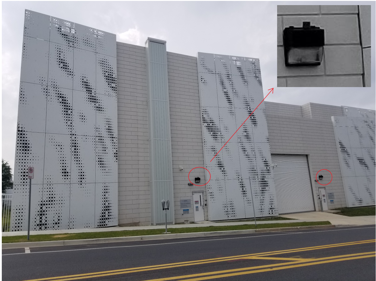
Photograph of Pepco's White Flint substation at 11650 Nebel St with "wall pack" fixtures
