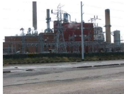
Prairie Creek Generating Station. Photo by Elwood Garlock.
