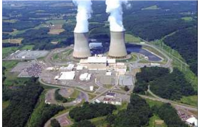
Cooling towers at a nuclear power plant. Photo courtesy Nuclear Regulatory Commission
