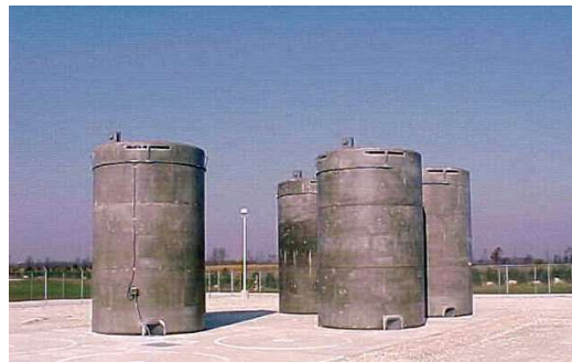
Spent fuel dry cask storage. Photo courtesy Nuclear Regulatory Commission
