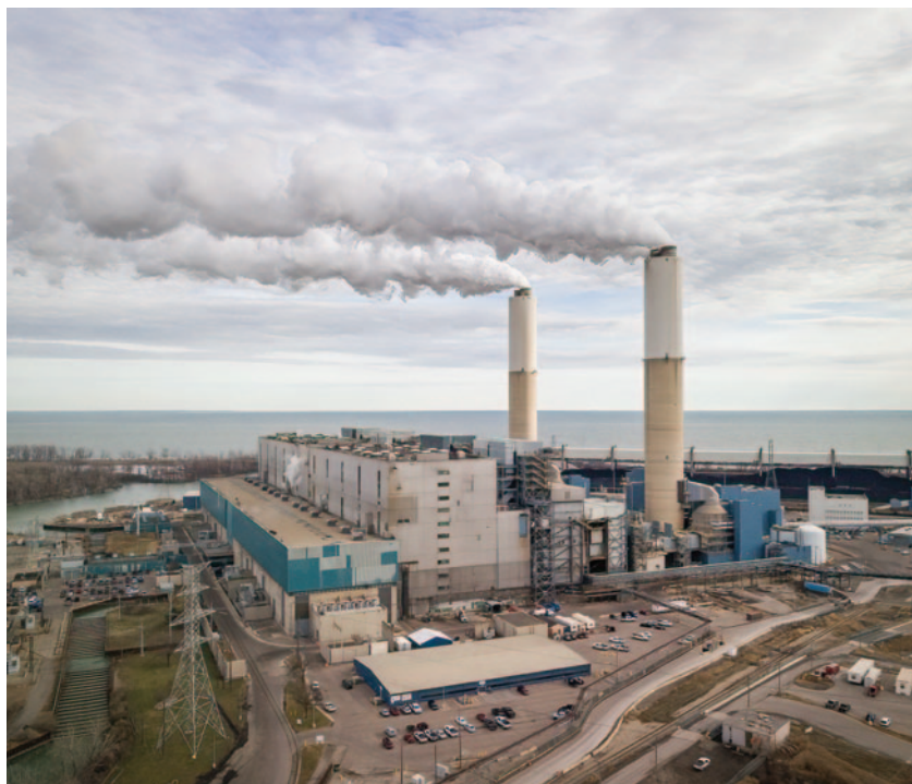
The DTE Monroe Coal Plant is scheduled to close in 2028.
